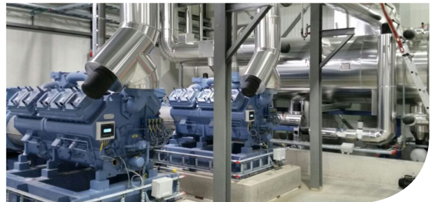
Heat pump systems
