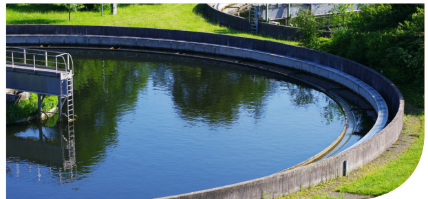
Water and waste water treatment
