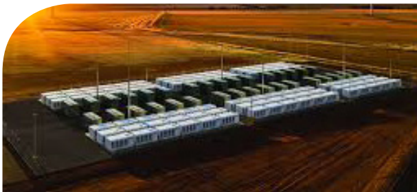
Energy and power
